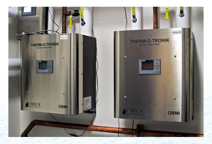
**NOTICE:** The **THERM-O-TRONIK** should not be the last hot water supply device for users applications. At the point of usage an Anti-burn cartridge is mandatory.
